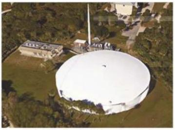
As is common with many water utilities, Punta Gorda was having difficulty maintaining optimal chlorine residuals for water disinfection in their distribution system. After pursuing common operational strategies such as tank flushing, operating at lower tank levels to reduce water age and distribution line flushing, the utility staff decided to employ a Tank Shark® mixing system in the larger 2 MG Punta Gorda Isles tank.
